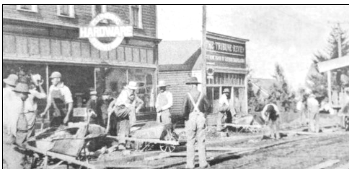
This 1917 photo shows the original Tribune-Review building at 312 Main St. It sat across the alley from the Edmonds Hardware Store. (Photo courtesy Edmonds Historical Museum)
