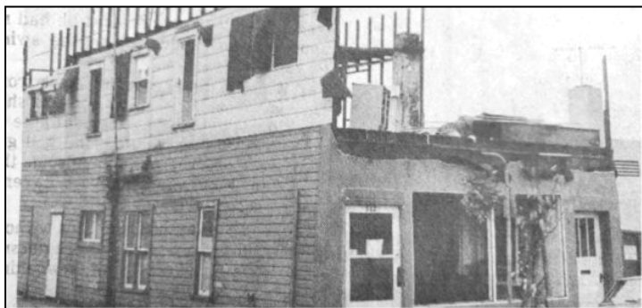
1976 demolition of the 1908 Tribune-Review building. (Photo courtesy Edmonds Historical Museum)
